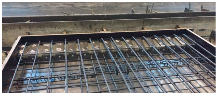
Shuttering with floor slab support profile
