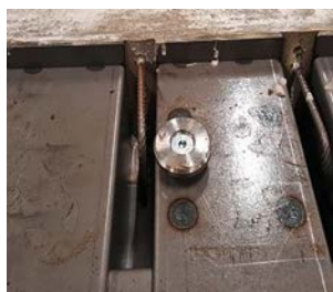
Shuttering with shear key and reinforcement penetration and finished element
